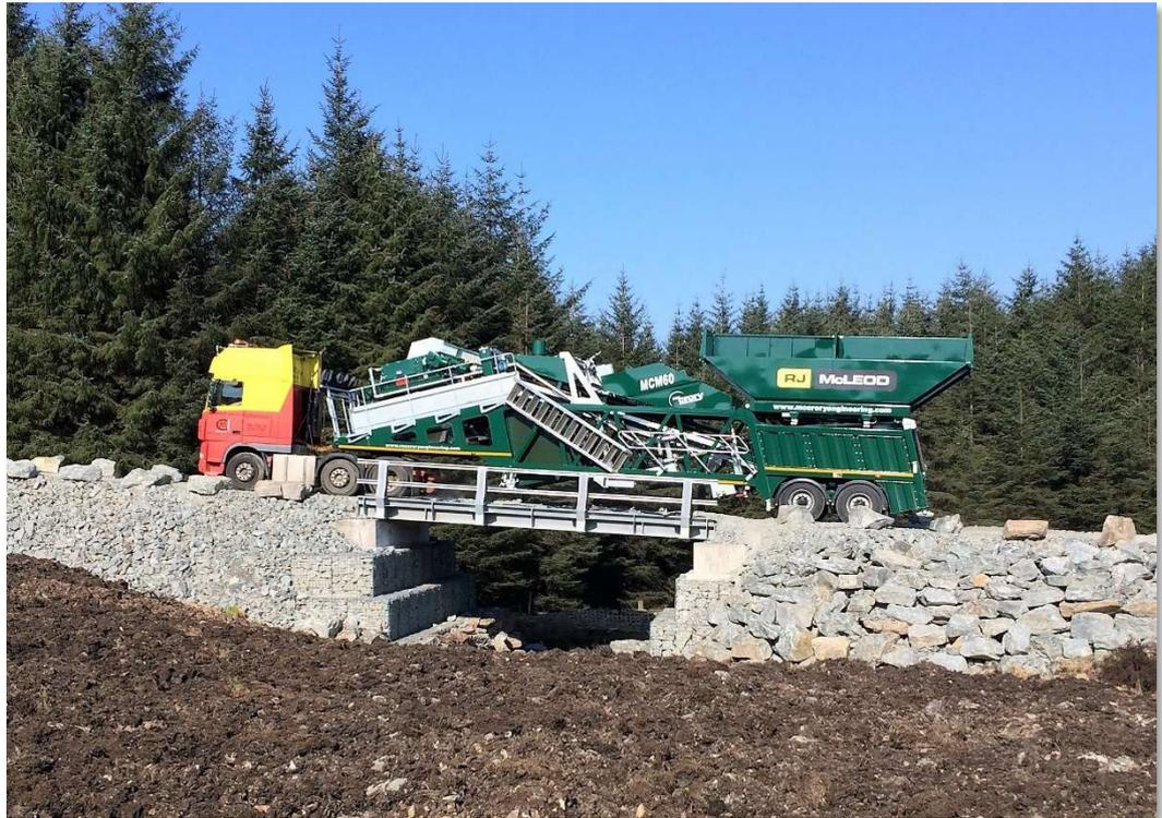
All bridges were single span - two were 8.9m long with a 4.5m roadway and the largest was 11.9m long with a 6.9m roadway.
